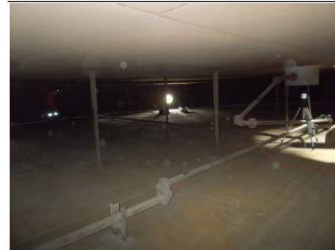
Photograph 2: Tank bottom overview.
