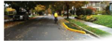
Carb Extension Bioswale Retrofit, PORTLAND, OR
