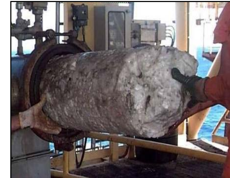
Block of methane hydrate obstructing pipeline
