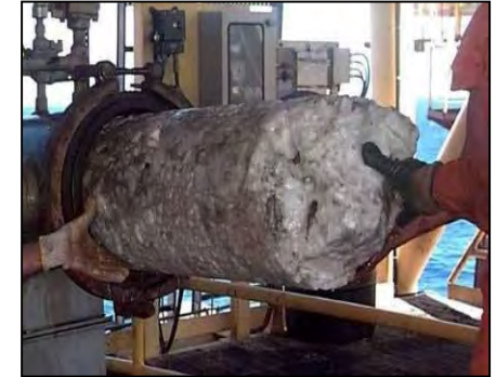
Block of methane hydrate obstructing pipeline
