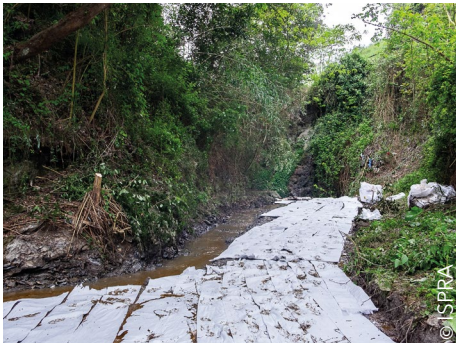
Protection of a working area with sorbent sheets
