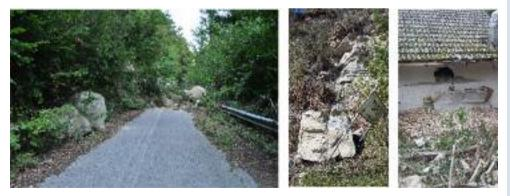
Figure 2: Left: Collapse of blocks that interrupted the road between the Salaria and the village of Tufo (AP); Center: Block collapsed on a road sign at the entrance of Tufo; Right: Wall of a house in Capodacqua (AP) damaged by a block rolled from the overlying slope Source: ISPRA
