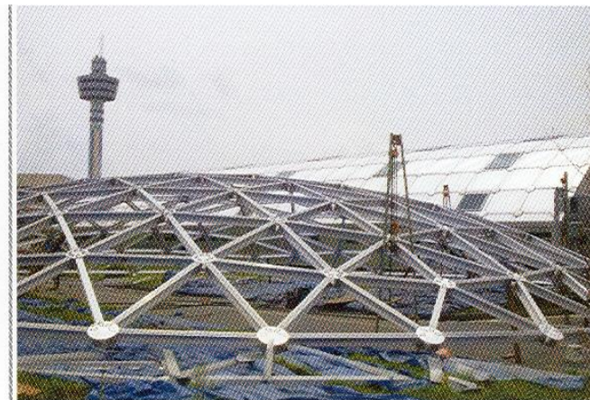
Assembling Main Frame
