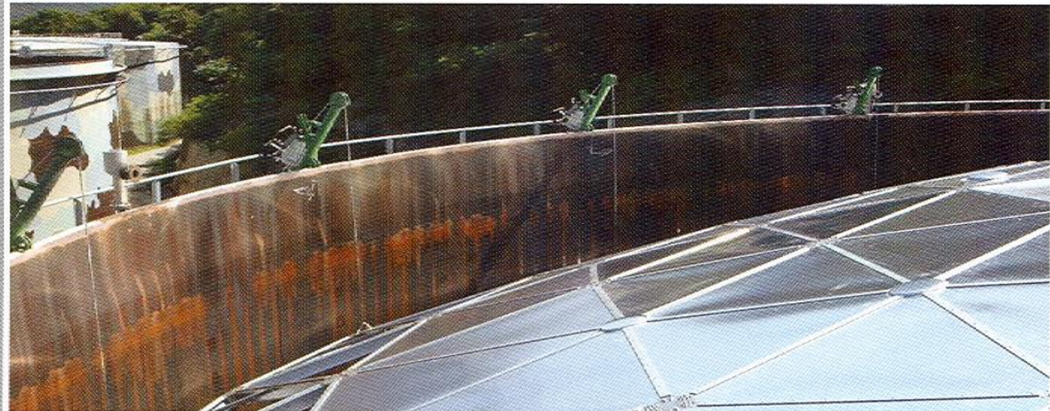
Special Lifting Systems for the Limited Space with no Ground Area for Dome Assembling Works
