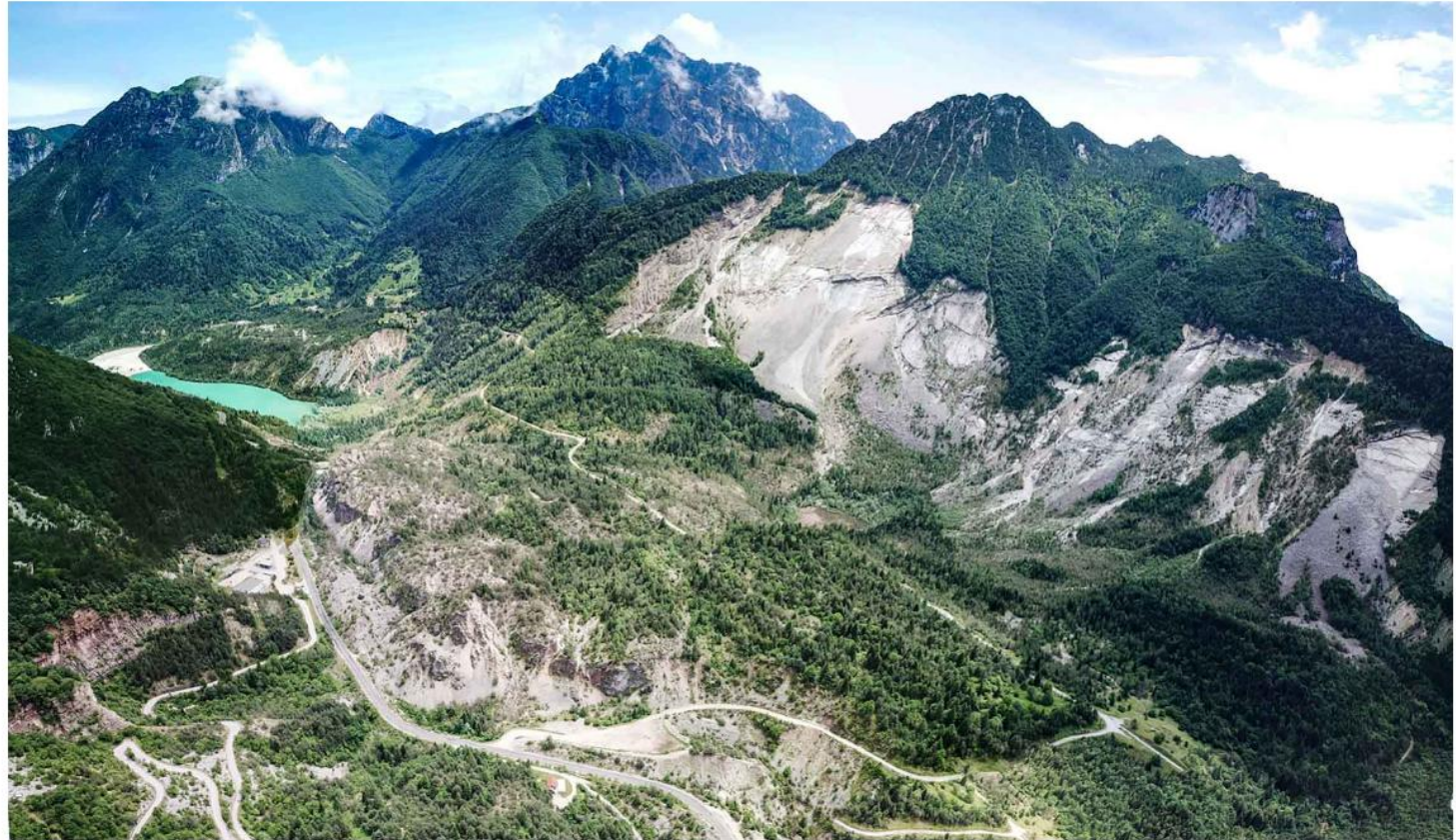
The extensive scarp and the huge body of the Vajont landslide detached from Mt. Toc (drone photo courtesy Monica Ghirotti).
