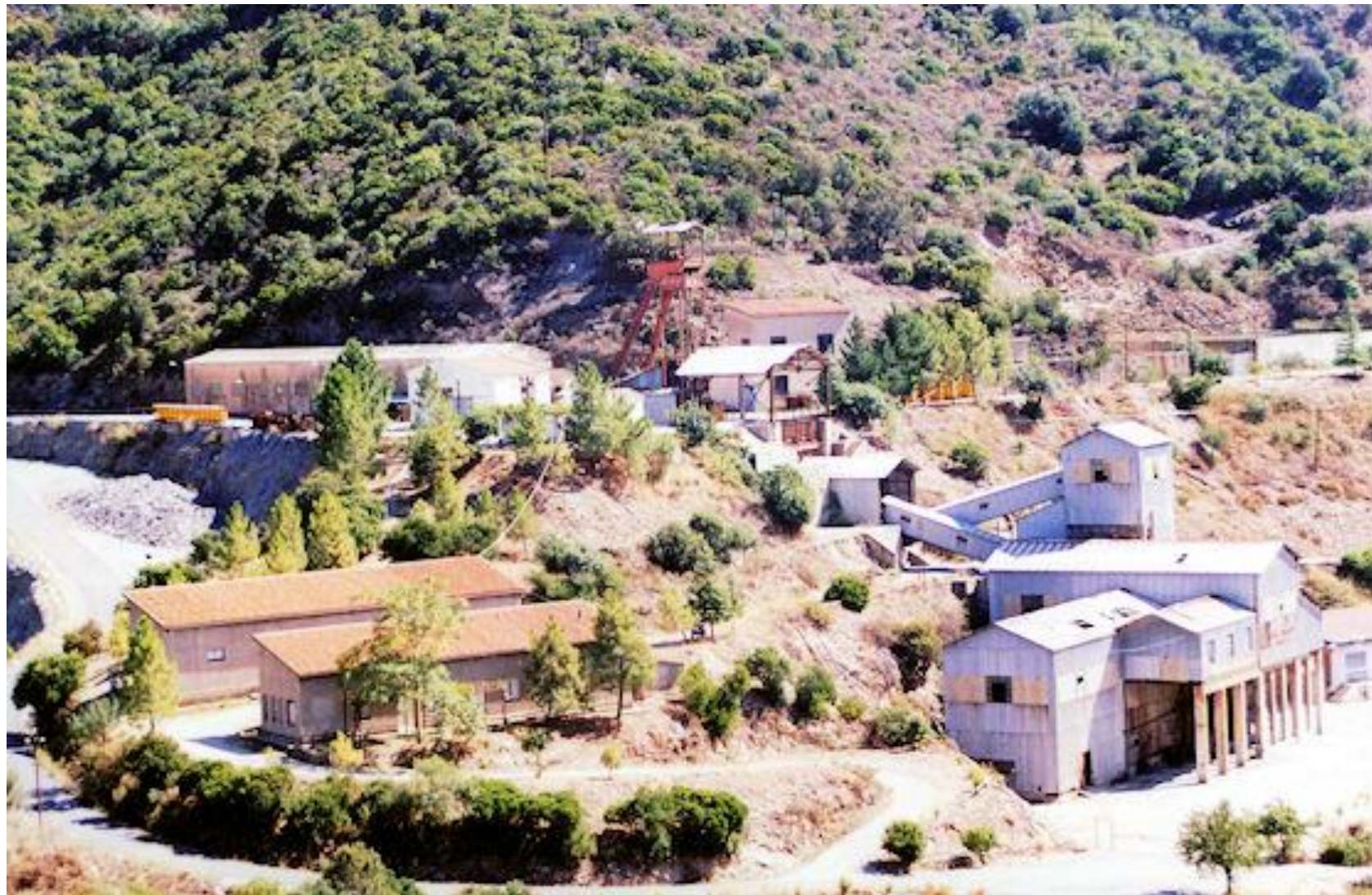
Aerial view of the Sos Enattos mining site, featuring the headframe, the workshops, and the processing (washing) plant built into the hillside.
