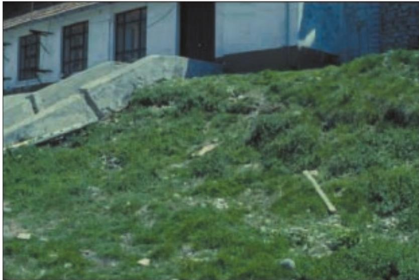
Fig. 8. A ground fracture cutting the stairs of the meteo station at Treviso
