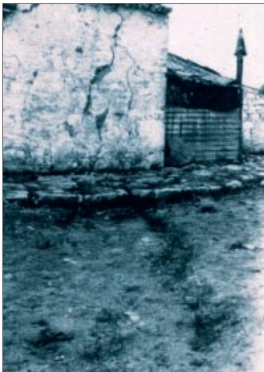
Fig. 2. Earthquake induced ground fracture cutting a house
