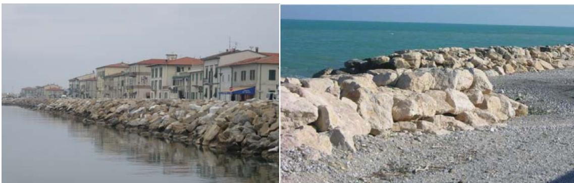
**Figure 1.1.3 – Some examples of riprap breakwaters: to the left, for a urban settlement protection (Photo by ISPRA); to the right, for a shoreline protection (APAT, 2007).**
