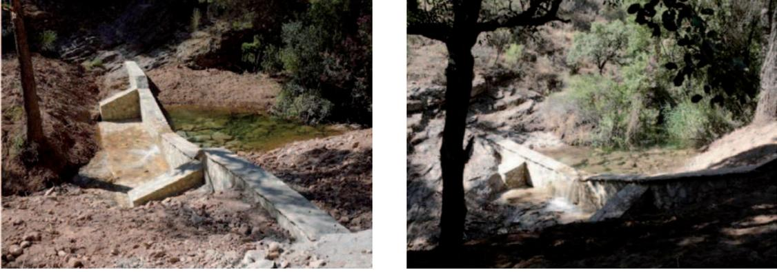
Figure 7. Temporary dikes installed to prevent the spread of the red crayfish (*Procambarus clarkii*) in a river colonized by the native and endangered white-clawed crayfish (*Austropotamobius pallipes*)
