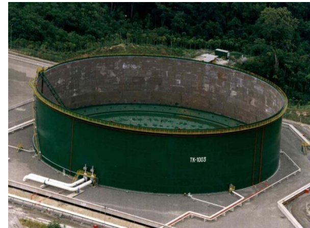
Floating roof tanks
