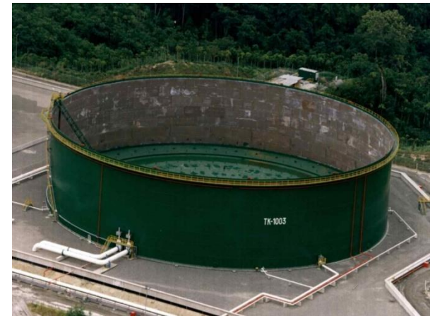
Floating roof tanks
