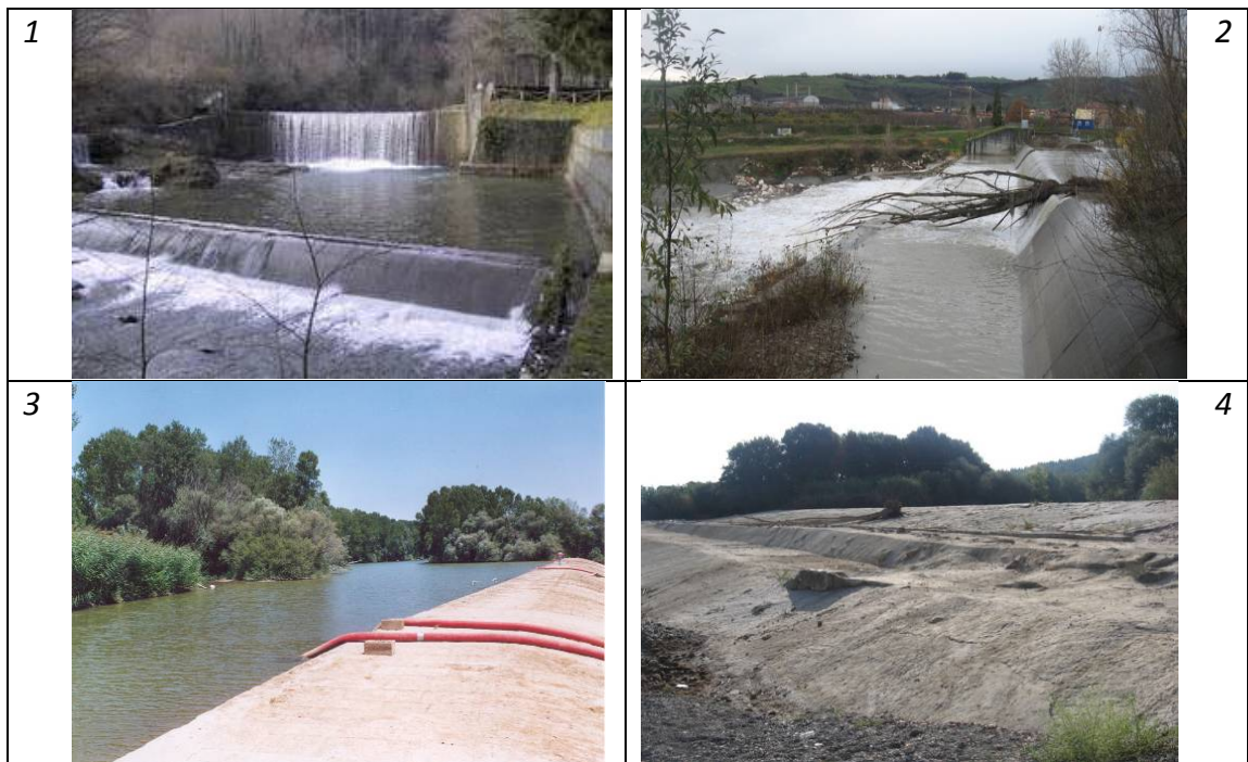
Figure A3. 40 Transversal structures of alteration of sediment discharges in hilly and lowland areas. (1) Consolidation check dam; (2) abstraction weir; (3) not filled abstraction weir; (4) filled abstraction weir.
