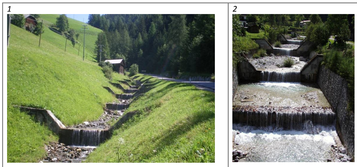
Figure A3. 46 Cases with very high density of transversal structures: An additional score of 6 or 12 (depending on the density) is applied.
